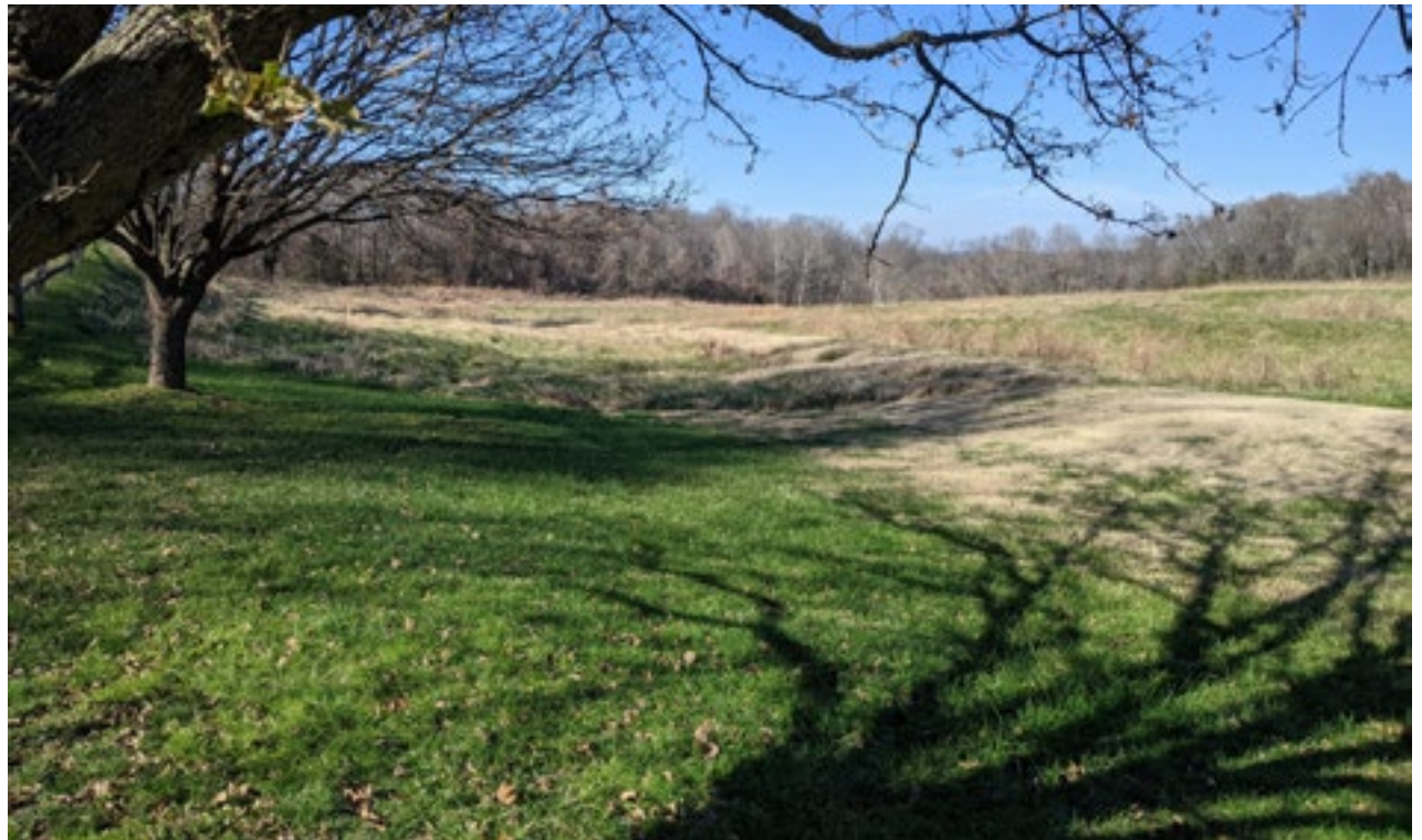
View of the Jefferson Park landfill from parking lot in Jefferson Park
