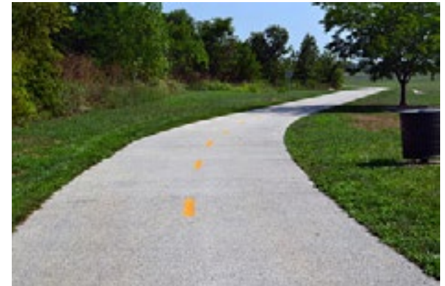
PerVIOUS hardscape used on a trail that will allow stormwater to infiltrate into the ground Source: perviouspavement.org
